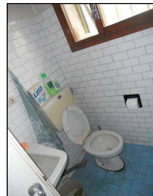
Piano Terra bagno
