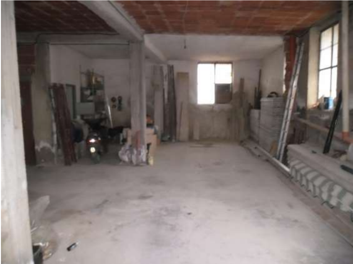
Figura 5 - Piano Terra (Garage)
