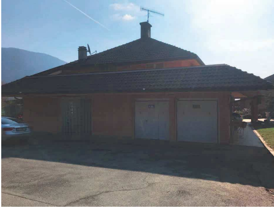
FG. 40, PARTICELLA 467, SUB. 5
