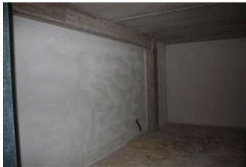
vista interna garage piano seminterrato sub 18
