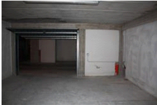
vista interna garage piano seminterrato sub 14
