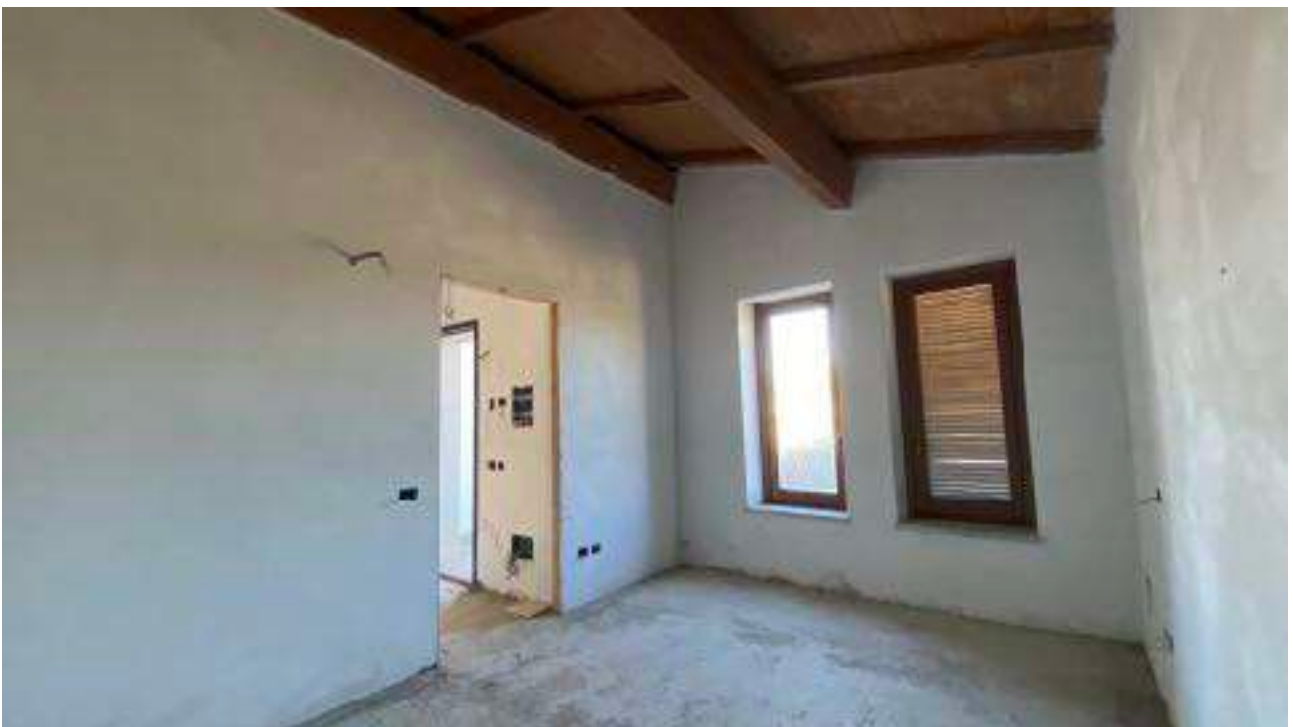
Villino bifamiliare sub 297 _ Camera
