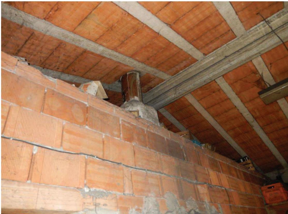
**PARTICOLARE COSTRUTTIVO: SOLAI E CAMINO A TETTO IN ACCIAIO (DIFFORME)**
