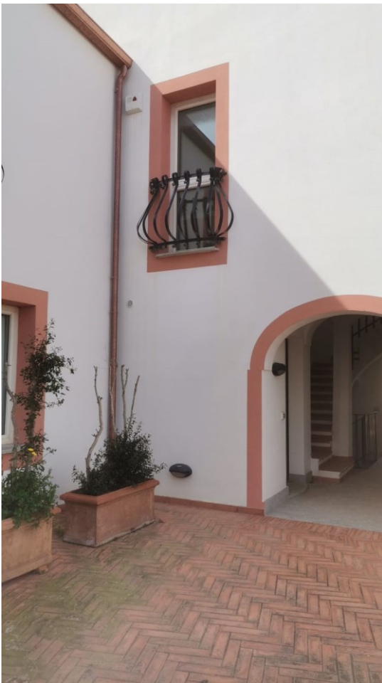
FIGURE 6: A) BALCONE IMMOBILE IN OGGETTO
