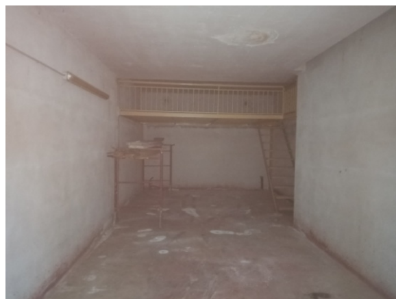
Interno garage Piano Interrato
