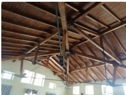
interni piano terra
