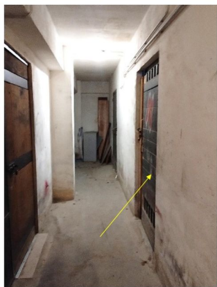
LOCALE CANTINA PIANO TERRA
