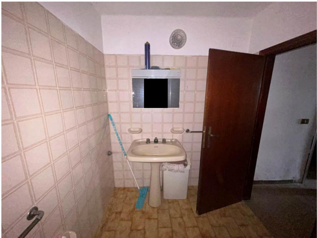
BAGNO (w.c.) – Piano Terra – vista 2
