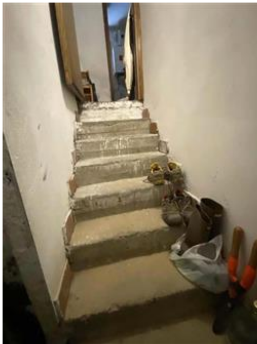
scala interna ps1-pt
