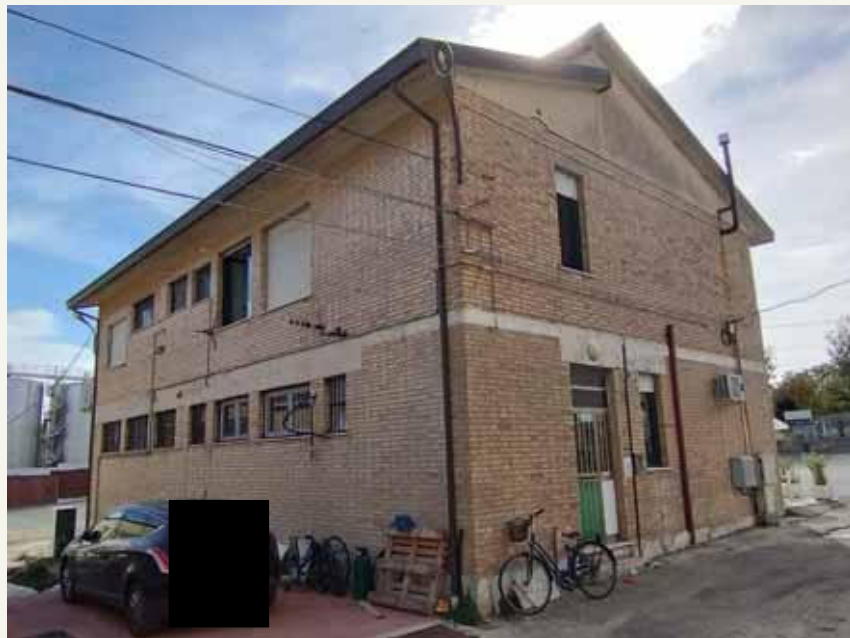
Lotto 8 – Lotto 9 – Lotto 10 – LOTTO 11: esterni
