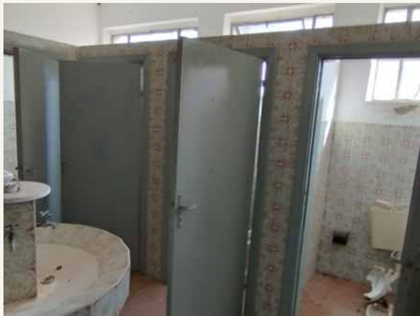
Lotto 3 – p.lla 159 s 9: interni
