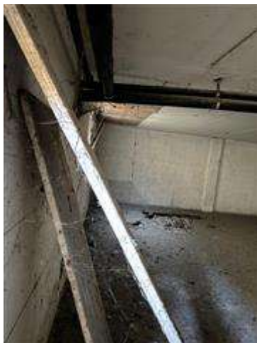
Rampa scale demolita
