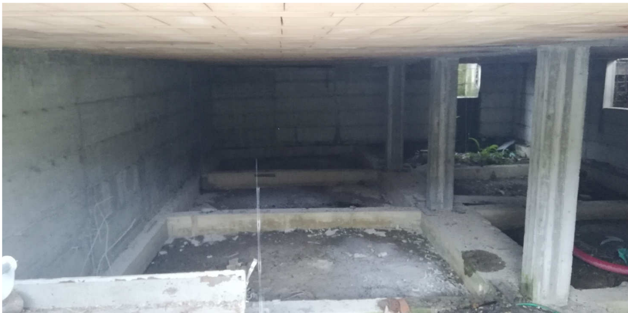
7) Vista piano interrato
