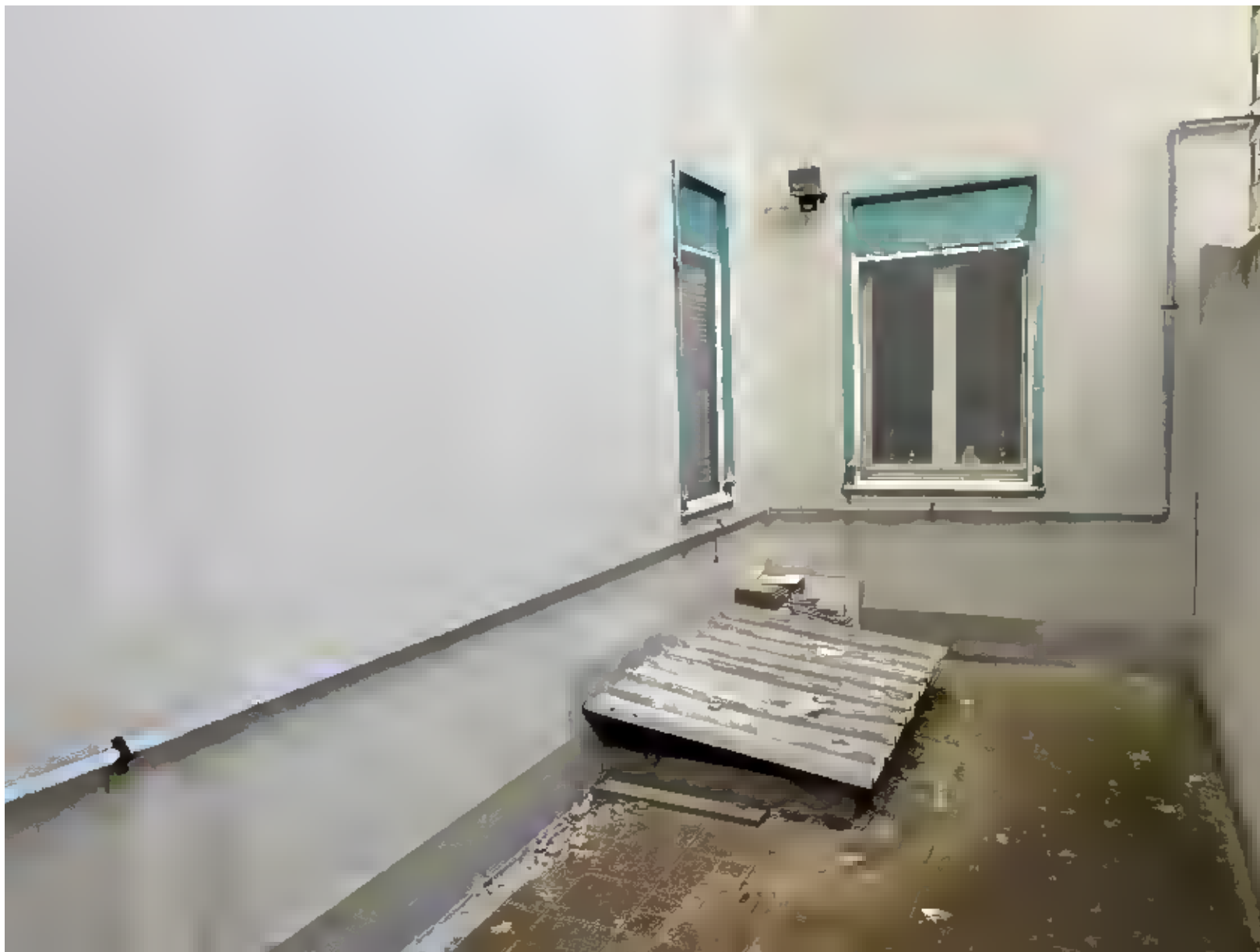
Figure 12 - vista area esterna
