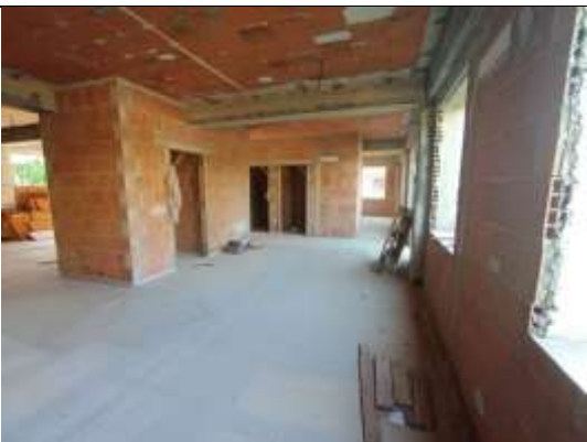
Piano seminterrato interno N-W
