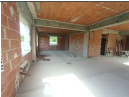
Piano seminterrato interno S-E
