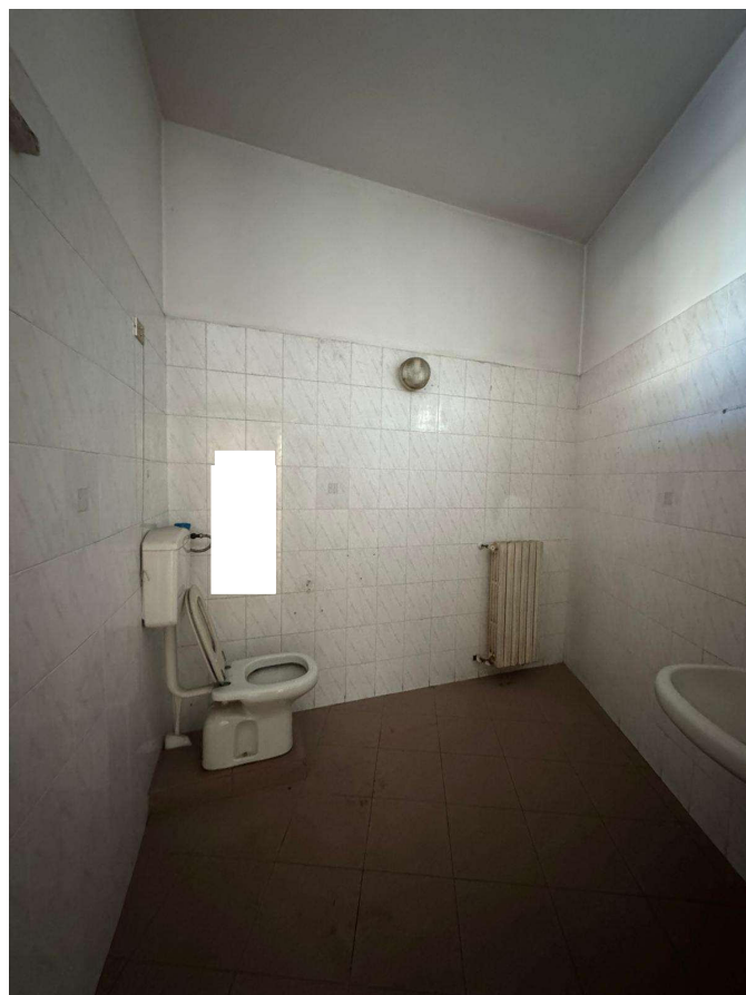
Piano terra: bagno
