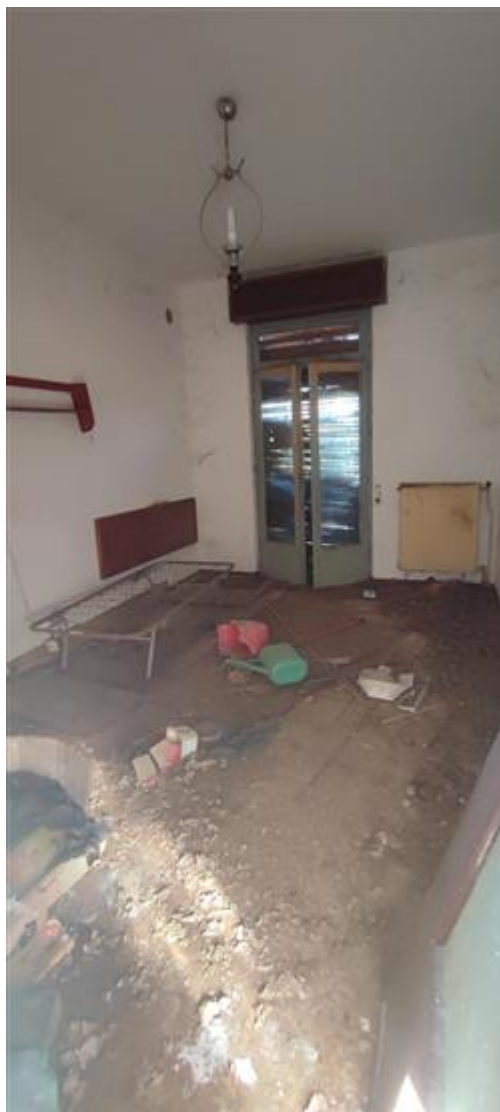
vista interna camera P1
