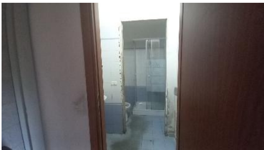
Wc piano terra
