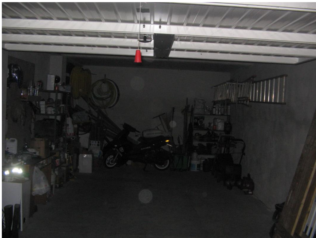
Interno box sub. 74 – piano interrato 2
