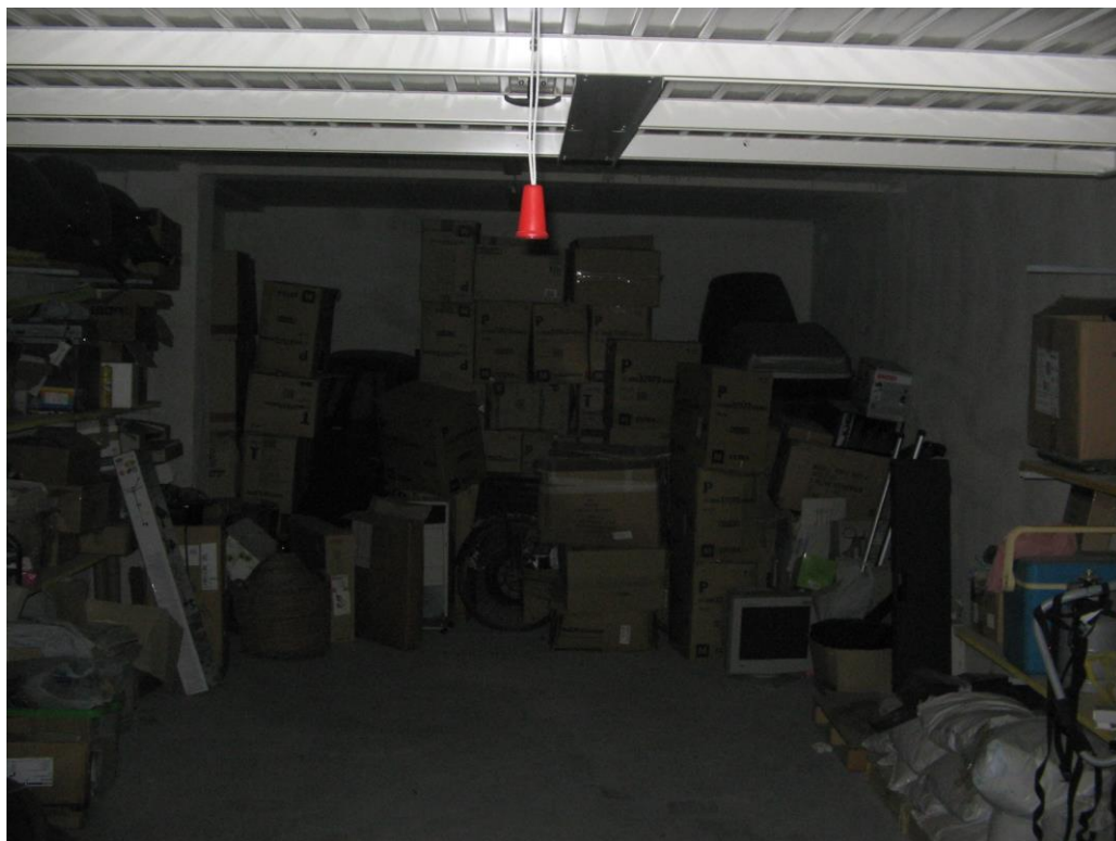
Box auto sub. 73 – piano interrato 2
