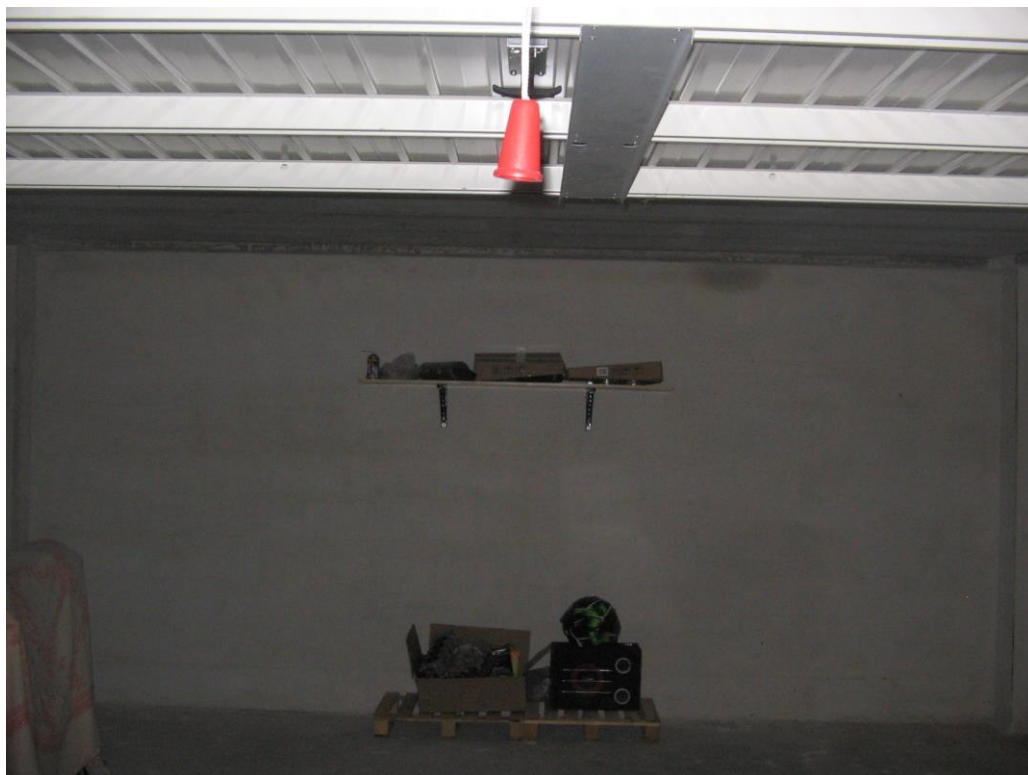
Interno box sub. 70 – piano interrato 2
