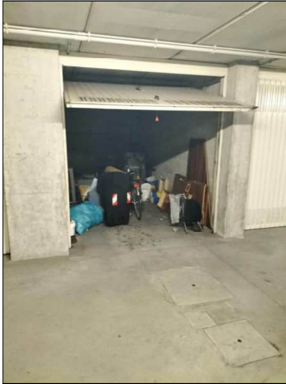
Vista garage piano interrato
