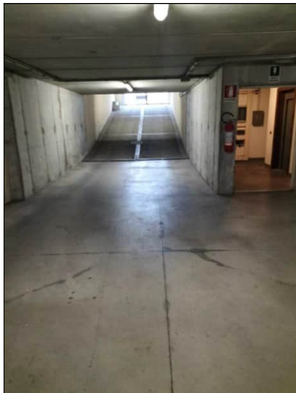
Rampa accesso garage piano interrato (Lotti 1 e 2)
