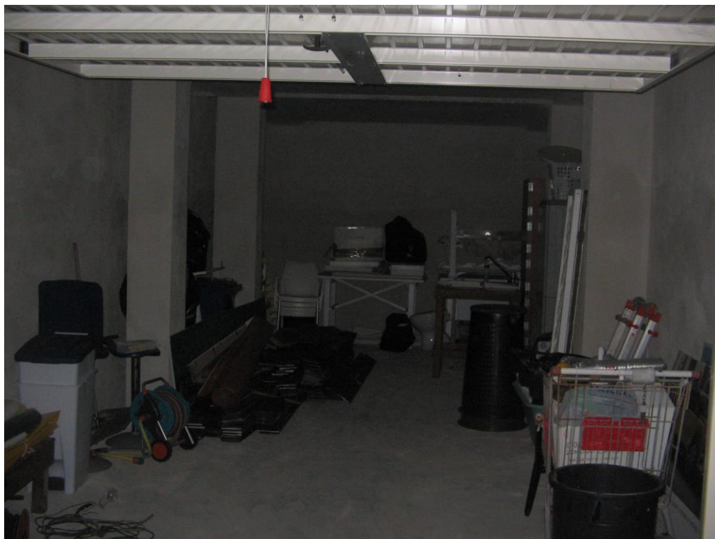
Interno box sub. 67 – piano interrato 2
