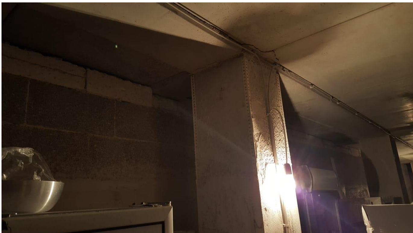
Interno box sub. 64 – piano interrato 2
