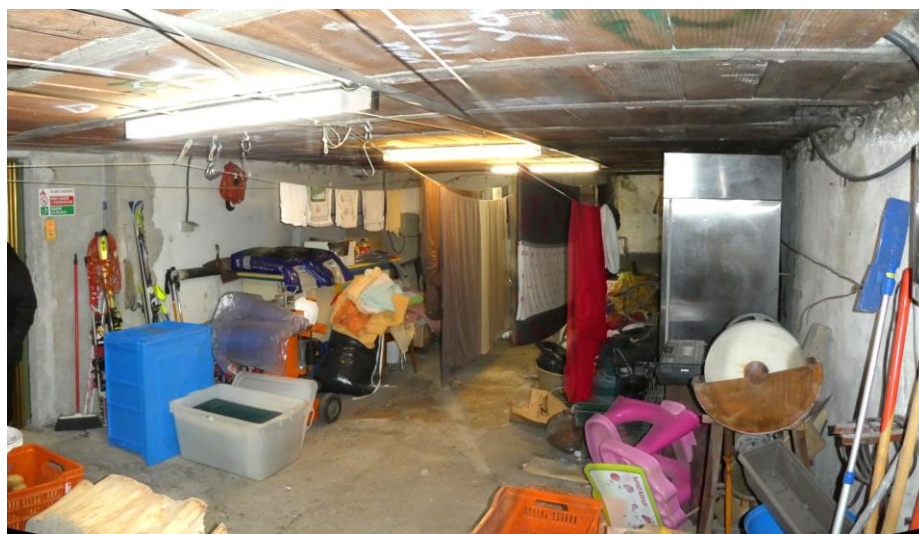
43. – locale Lavanderia – piano Interrato
