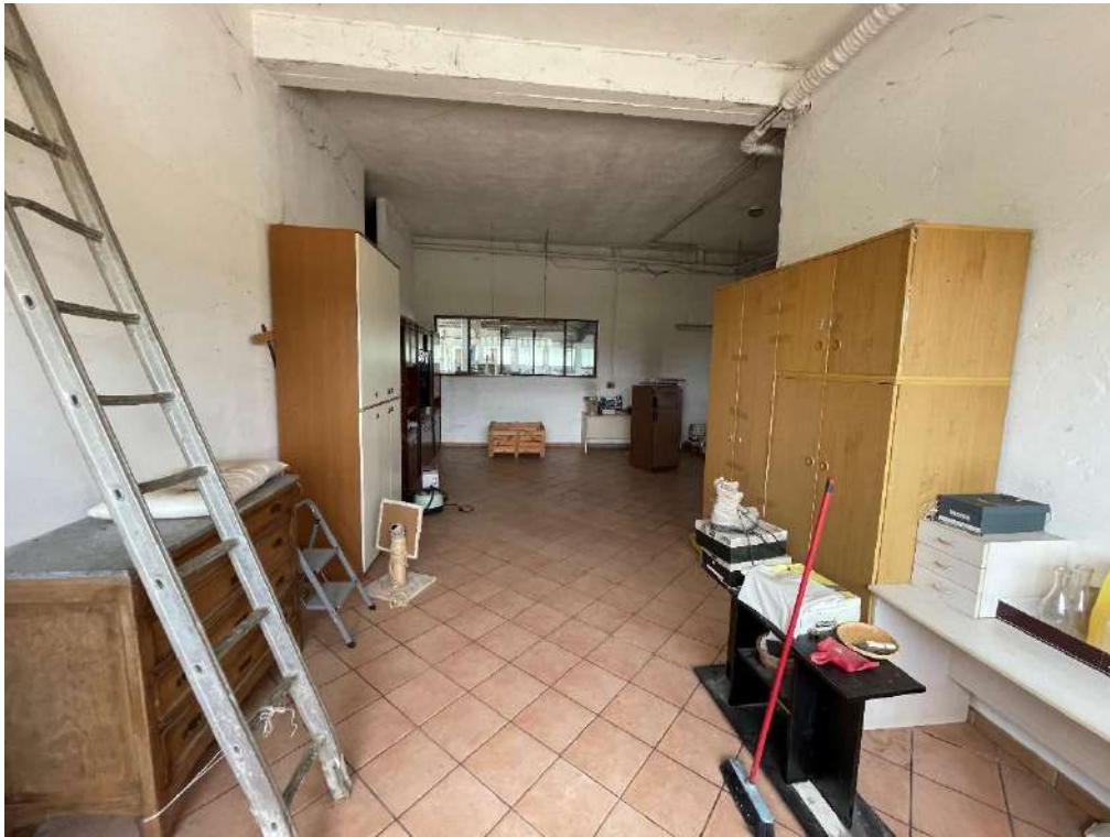
Piano Terra - Laboratorio - Sub.1 (foto 5)
