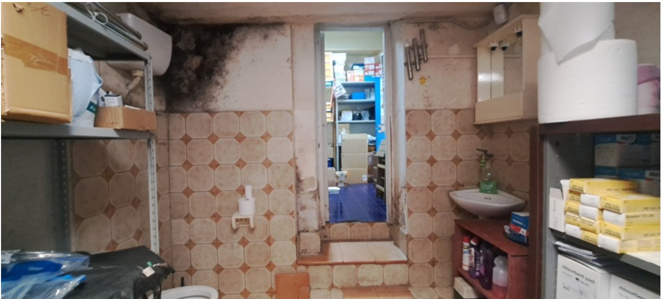
11 – LOCALE RETRO 2 WC
