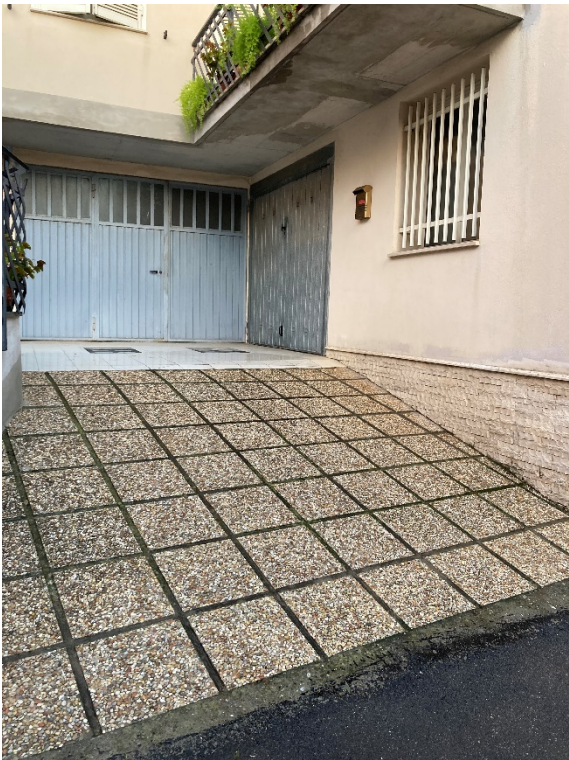
GARAGE - FG. 28 P.LLA 680 SUB. 9
