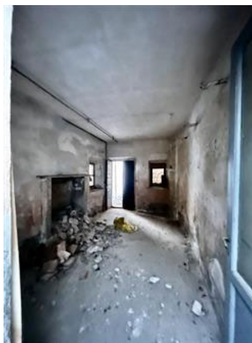
Locale al piano terra
