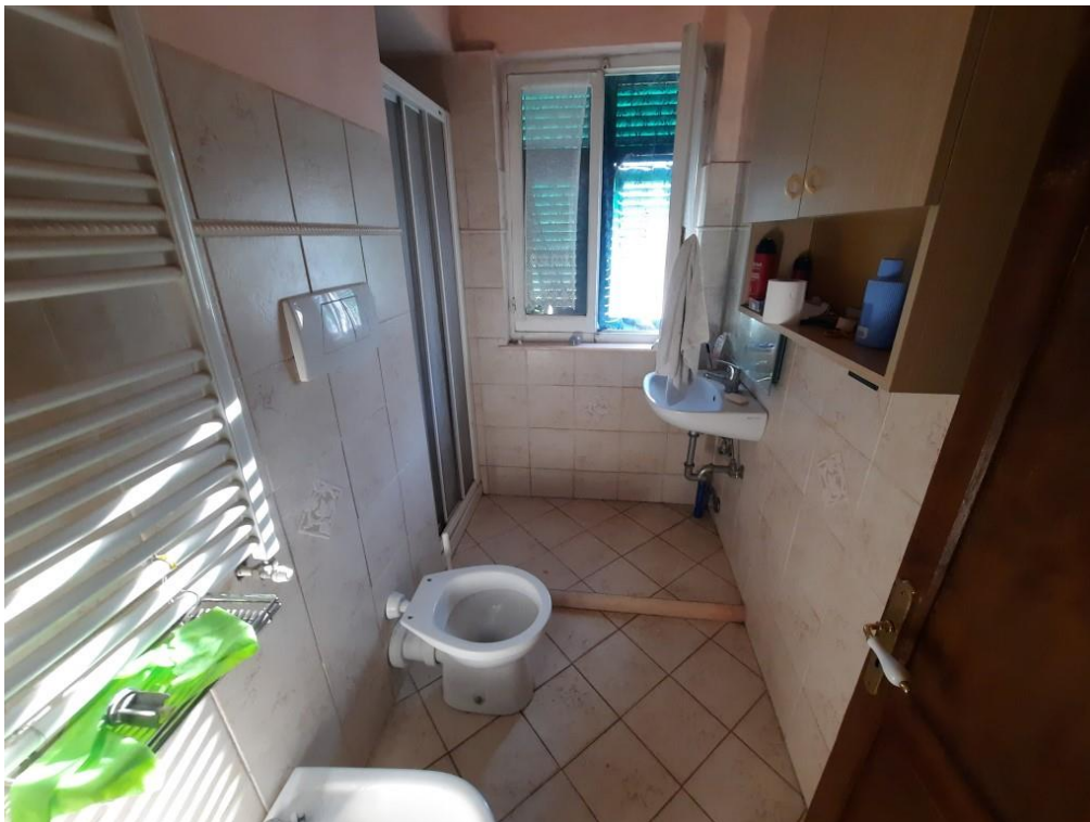
Figure 16– piano terra interno
