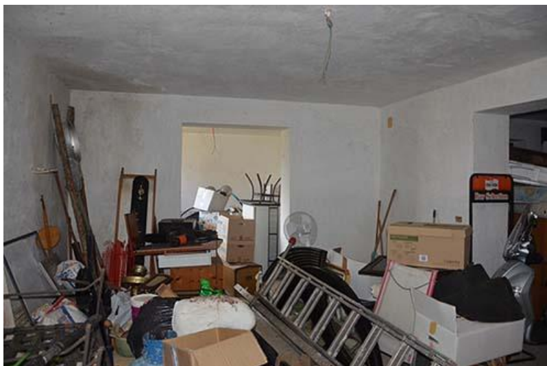
imm2.21: deposito (locale 2)
