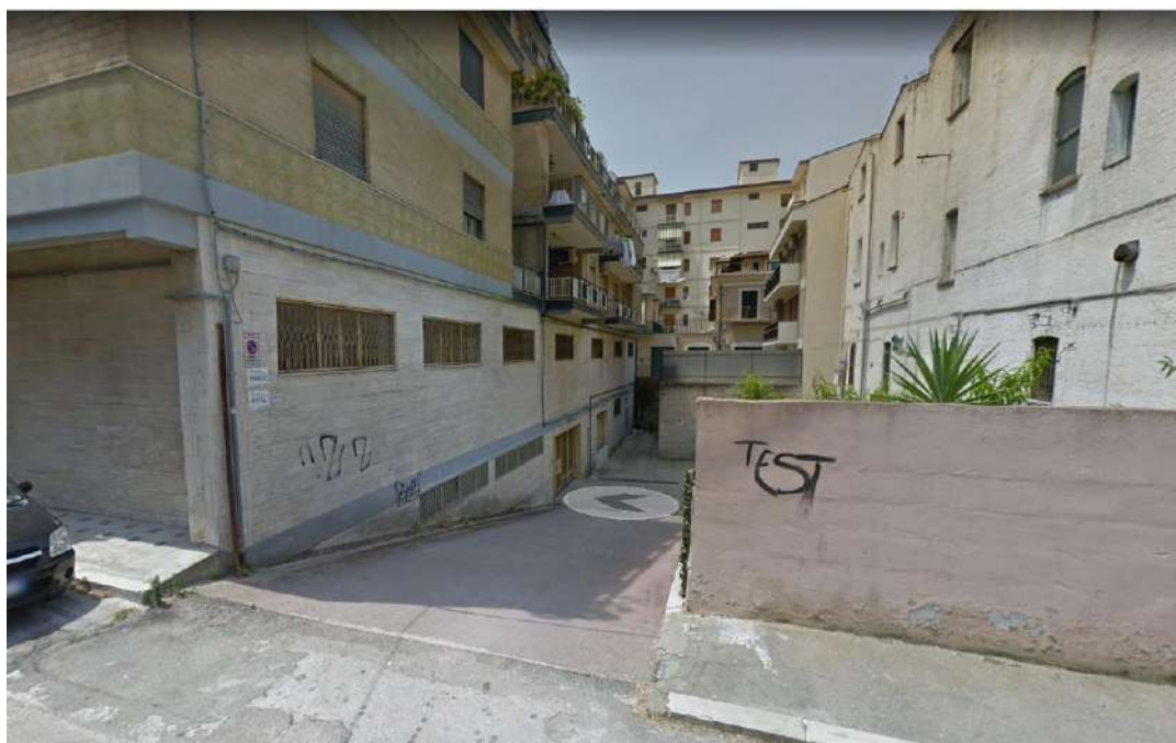
Figura 6: Dep.in Autorimessa condominiale, via Monte Santo, 3/A - San Severo (FG) – F.63 p.lla 797 sub.42 piano S1
