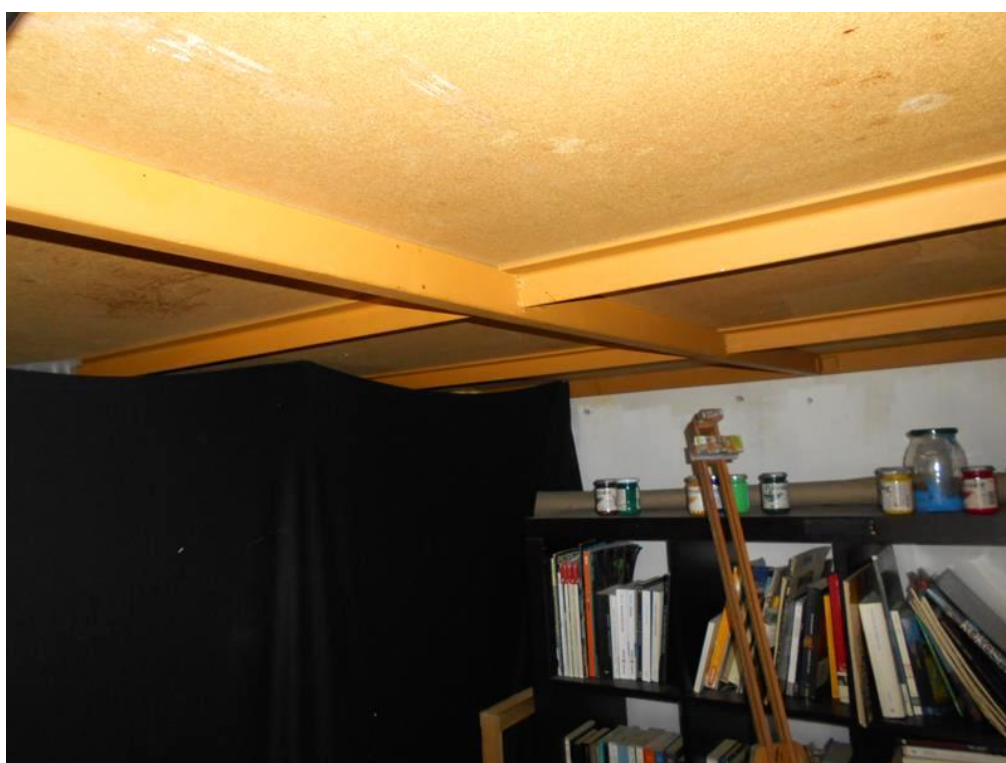
Foto 26- Locale garage al piano terra in NCEU al FL 2, P. LLA 1095, SUB 52
