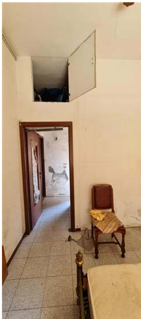
Camera piano terreno
