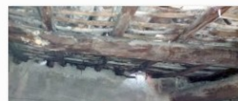
Deposit P1 Coperture.jpg
