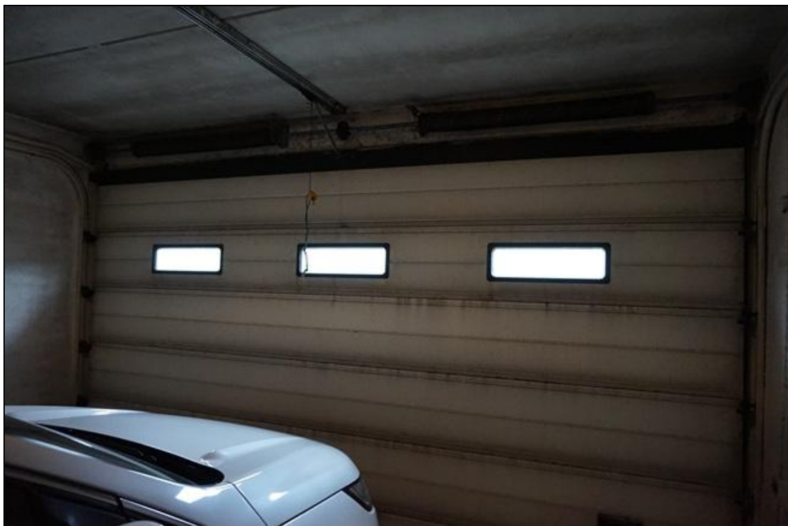
FOTO 37 – Piano interrato – Portone garage sub.45
