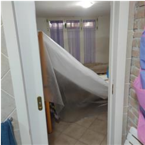
Interno Piano S1 sub 46
