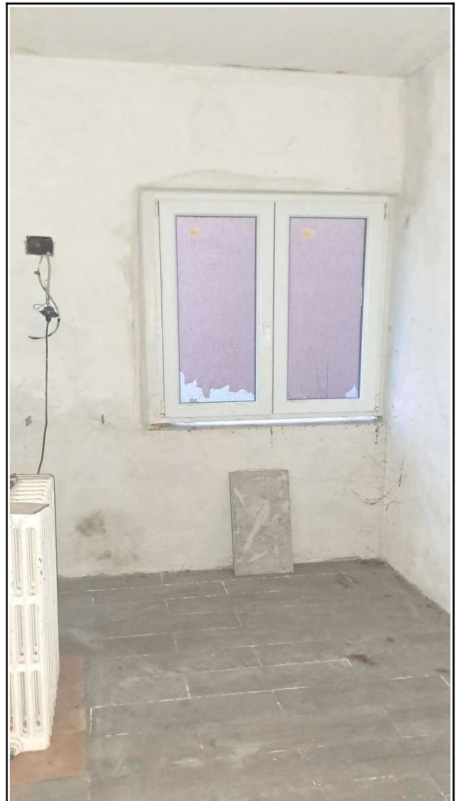
Camera 2 - Piano Terra
