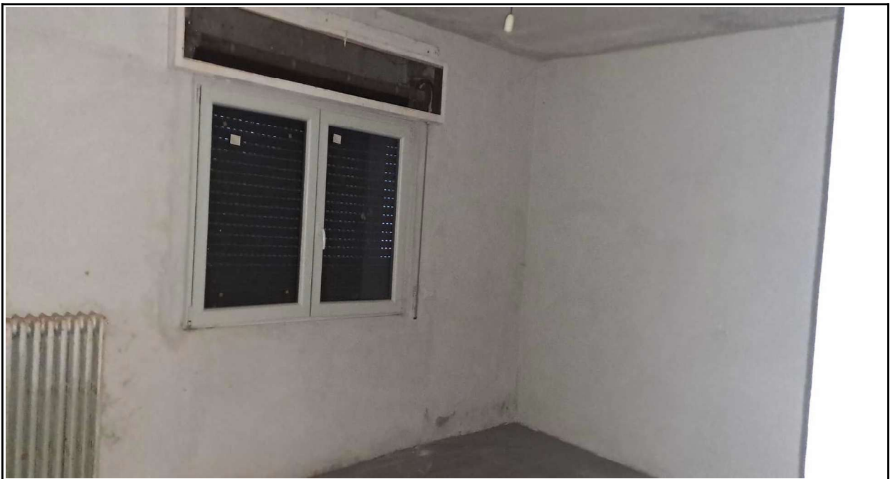
Camera 1 - Piano Terra
