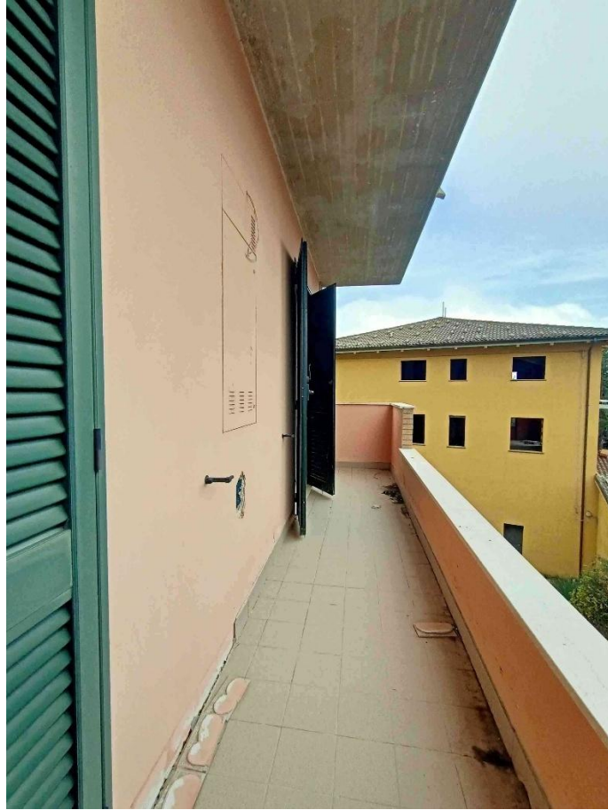
Foto 11: BALCONE SUB. 26 PIANO 1
