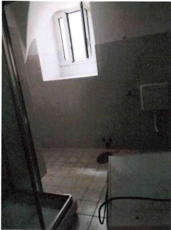
BAGNO PIANO TERRA
