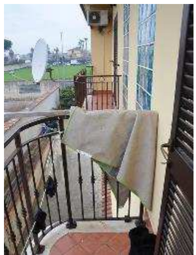
_camera e balcone – sub. 2
