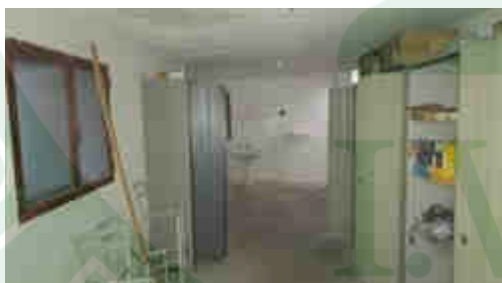
Locale al piano seminterrato
