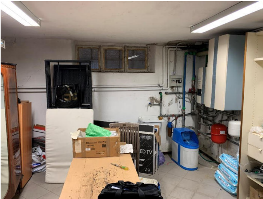
22 locale cantina piano seminterrato
