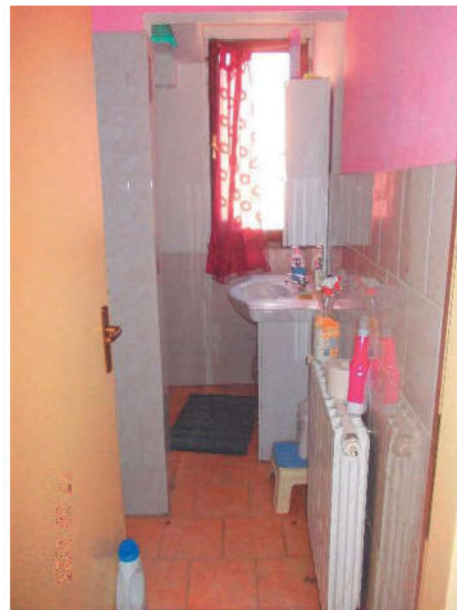
Vista locale bagno piano terra
