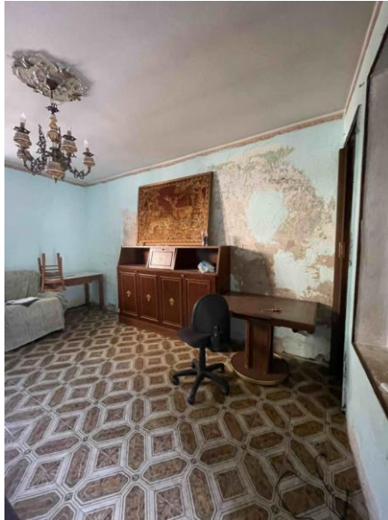
Locale al piano terra
