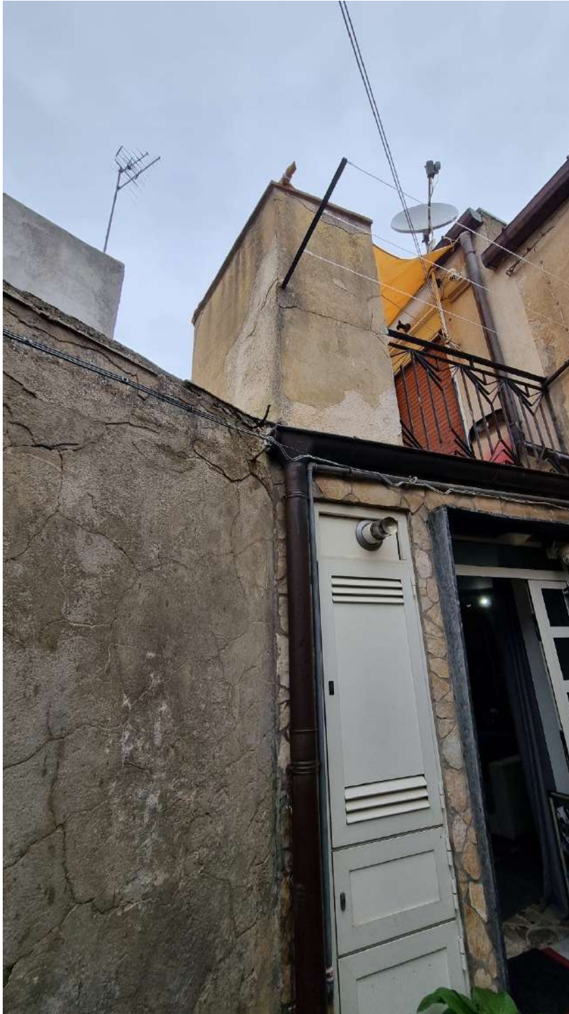
20251118_100819 – Esterno – Via San Sebastiano
