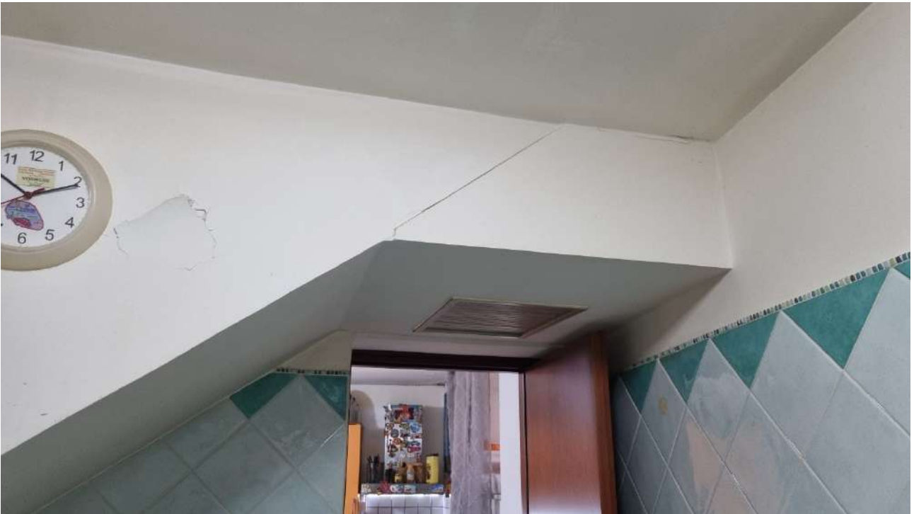
20251118_101034 – Piano Terra – W.c.
