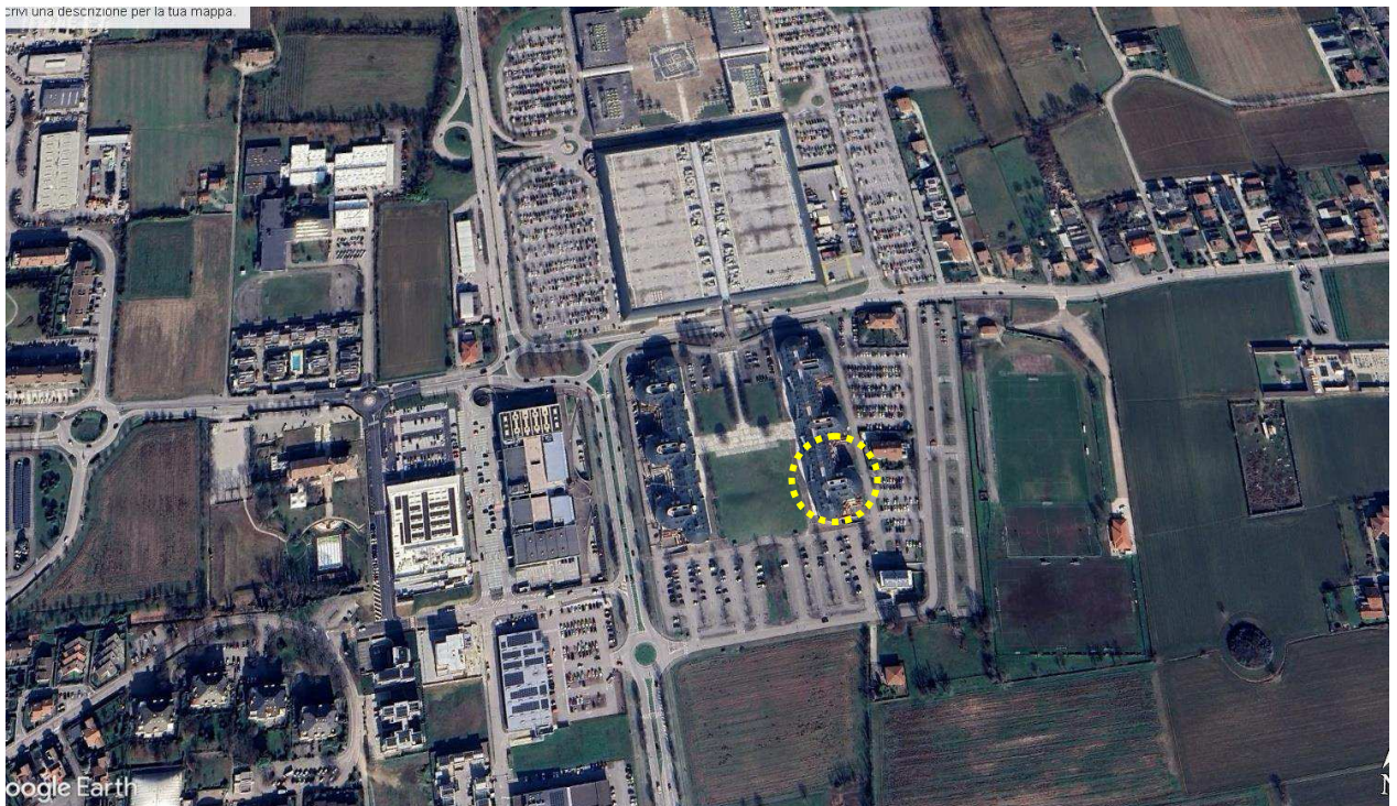
Ortofoto, Castel Franco Veneto, Condominio "Le Logge" scala F
