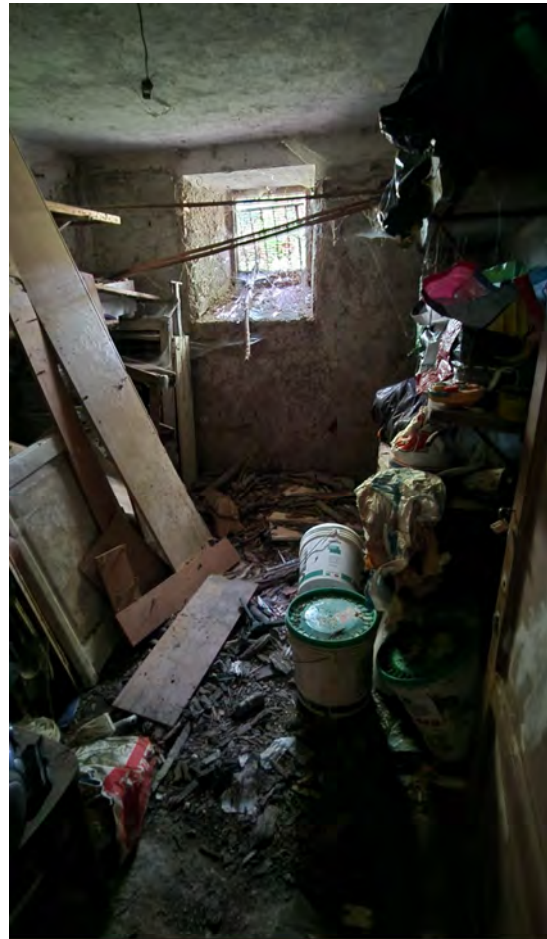
Cantina - Piano S1
